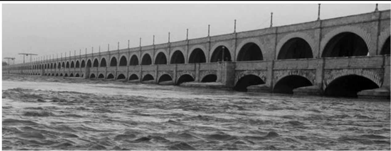
890. A view of Sukkur Barrage.
