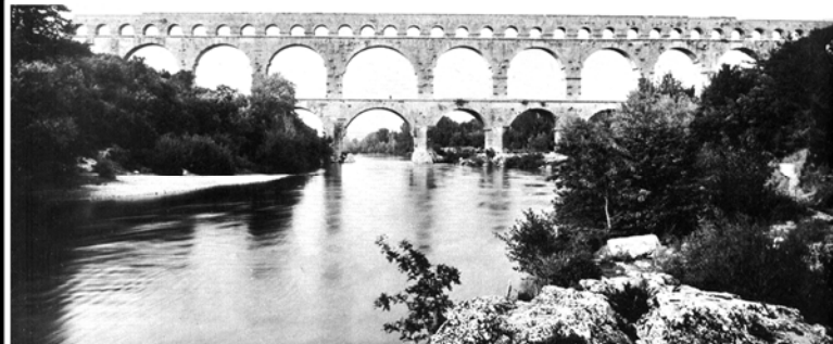
871. Pont du Gard near Orange. 1st century AD. Roman aqueduct constructoin, consisting of superimposed arches. compare with Sukkur Barrage (MWK).
